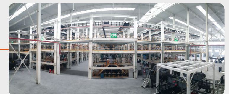
Threading, Air Pressure Test, and Anti-rust Treatment
